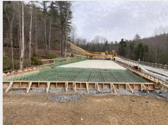
MC444- The bridge deck pour has been completed for phase 1.
