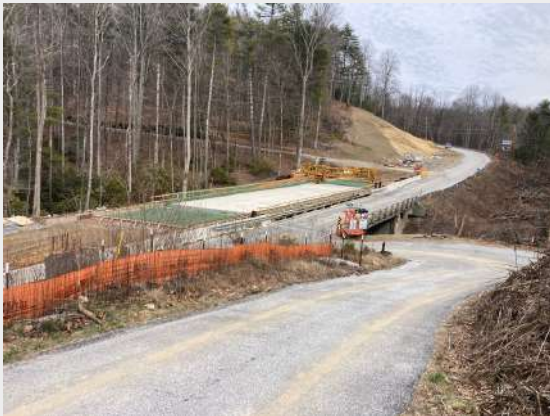
MC444- The bridge deck pour has been completed for phase 1.
